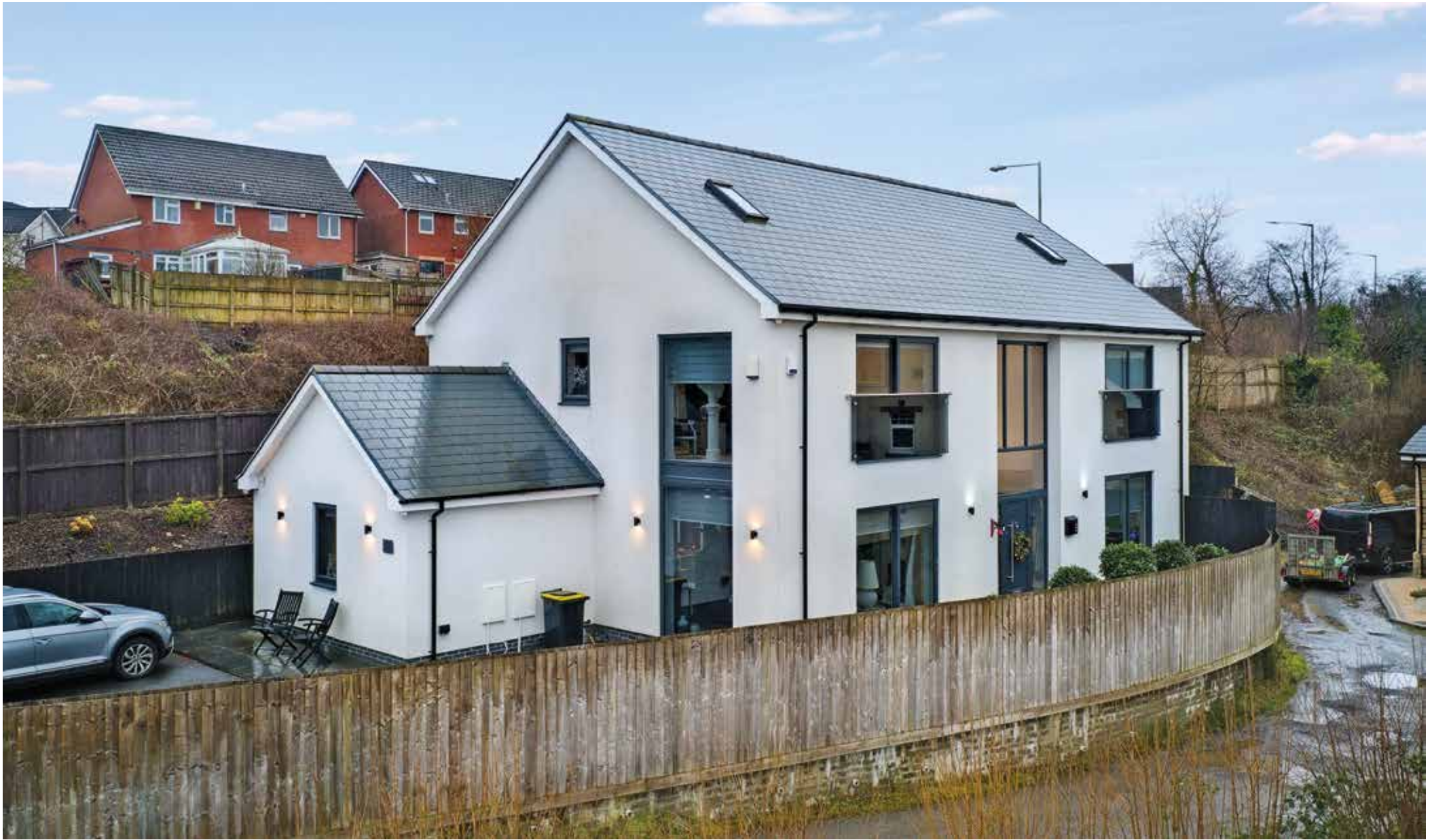
Bay Tree House Swansea Road | Merthyr Tydfil | CF48 1PB
